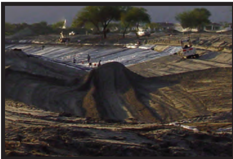
Construction of a 900 foot lake on the number nine fairway.
