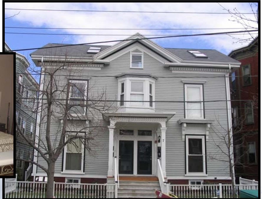
Exterior after renovation
