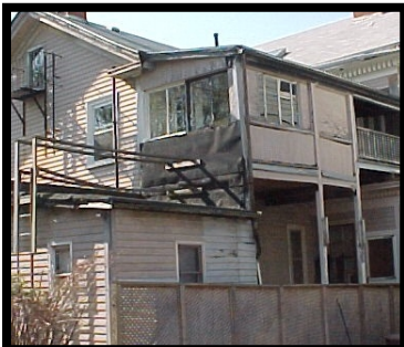
Exterior before renovation
